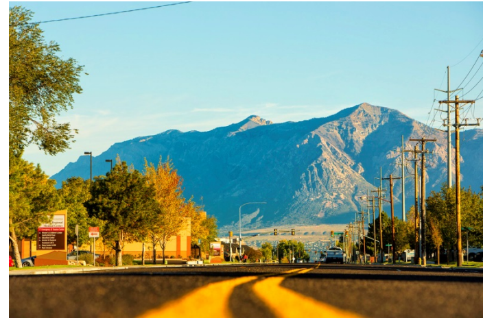
Image (left) Southeast Project Area - Adams Ave. between Washington Blvd. and 5600 South
