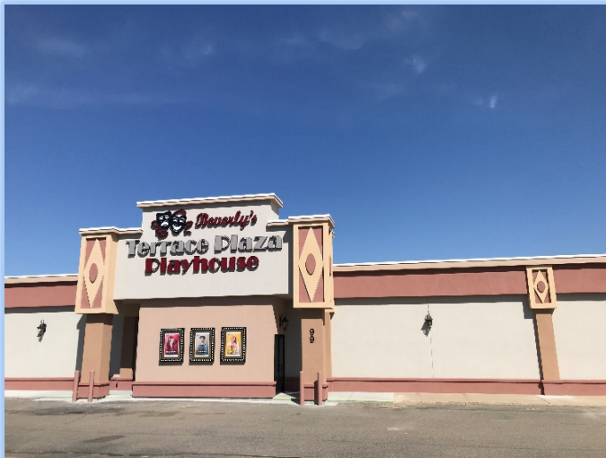
Image (above) CBD Project Area – Terrace Plaza Playhouse renovation
